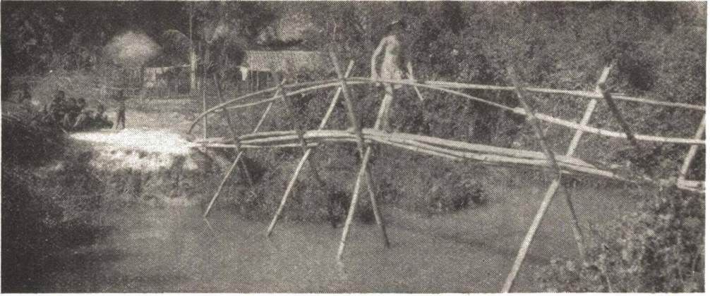
A primitive bamboo bridge in Burma.
